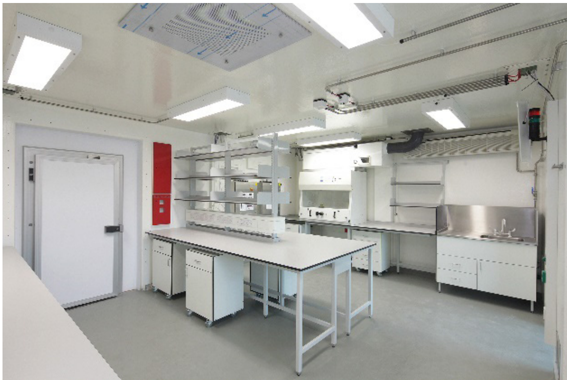
Copyright: Shepherd Construction.
